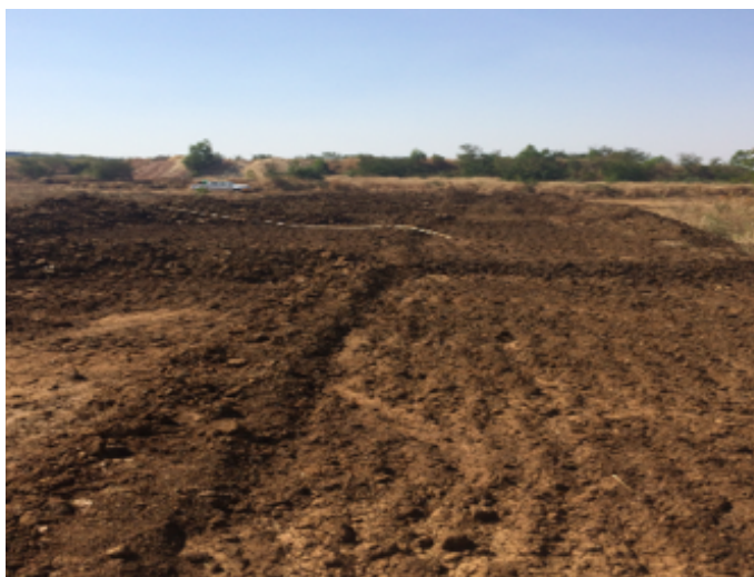
Removal of top soil not good for construction of lake bunds
