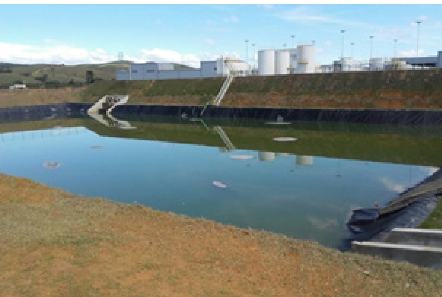
Itatiaia vehicle assembly plant – Rainwater balancing and abstraction pond for water reuse
