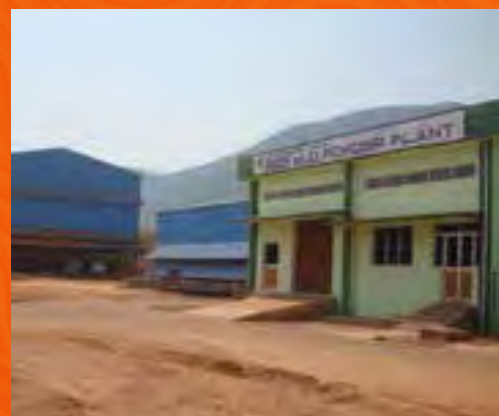
Red Mud Powder Plant at SSL – Lanjigarh
