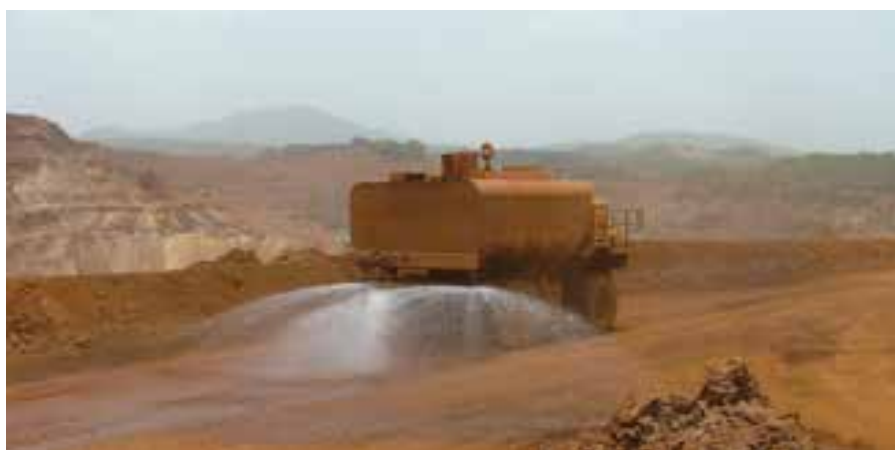
Dust suppression measures on haulage roads at HZL mine
