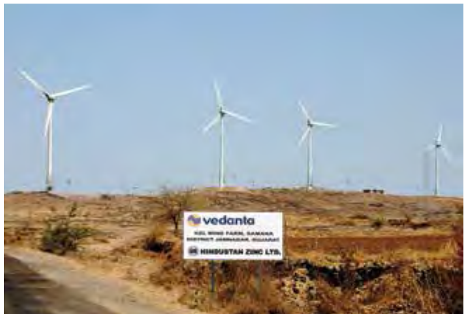
HZL operates around 273mw of wind turbine assets
