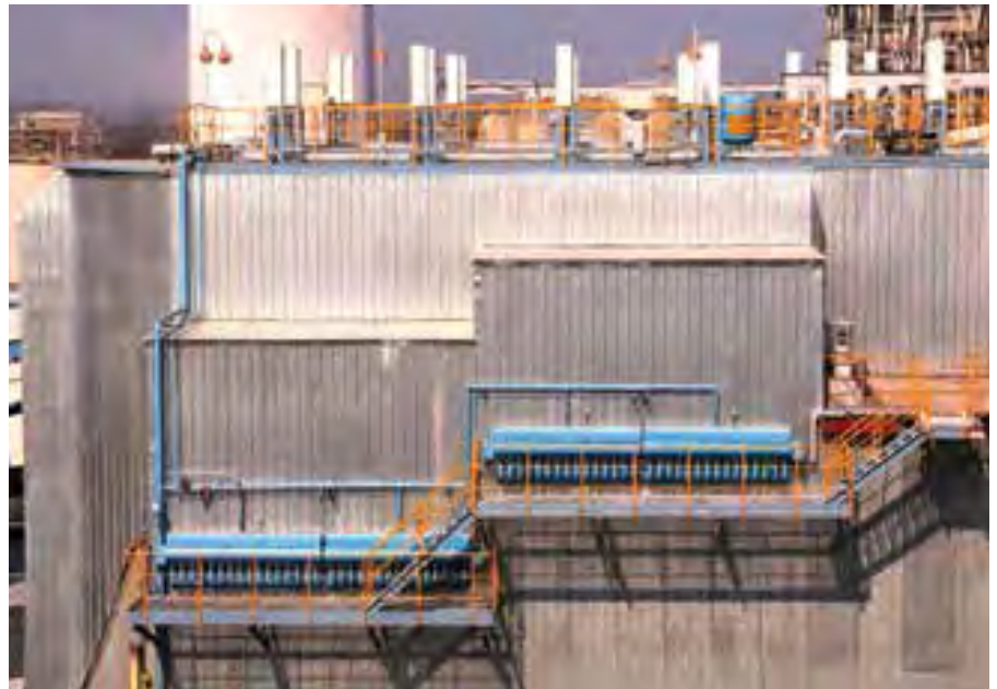
Hybridisation of ESPs with bag filters at SSL – Jharsuguda
