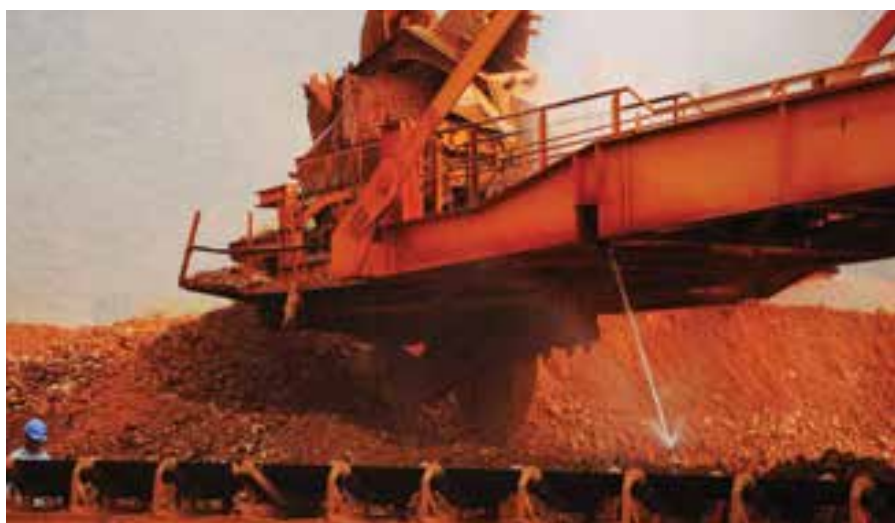
Water sprinkling system at Lanjigarh
