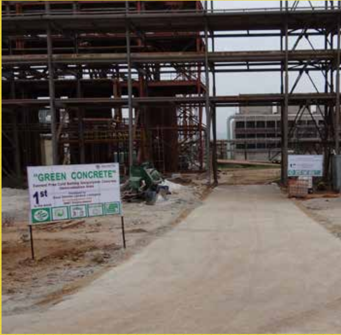
Road made of Cold-Setting Geopolymer Green Concrete at Vedanta Ltd. – Lanjigarh, India.
