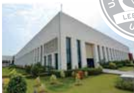
Green Factory, Vadodara
