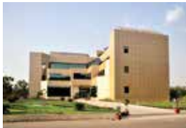
Administrative Building, LTSSHF, Hazira
