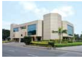
SBU Block (2nd floor), Hazira
