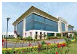
Administrative Building, Vadodara
