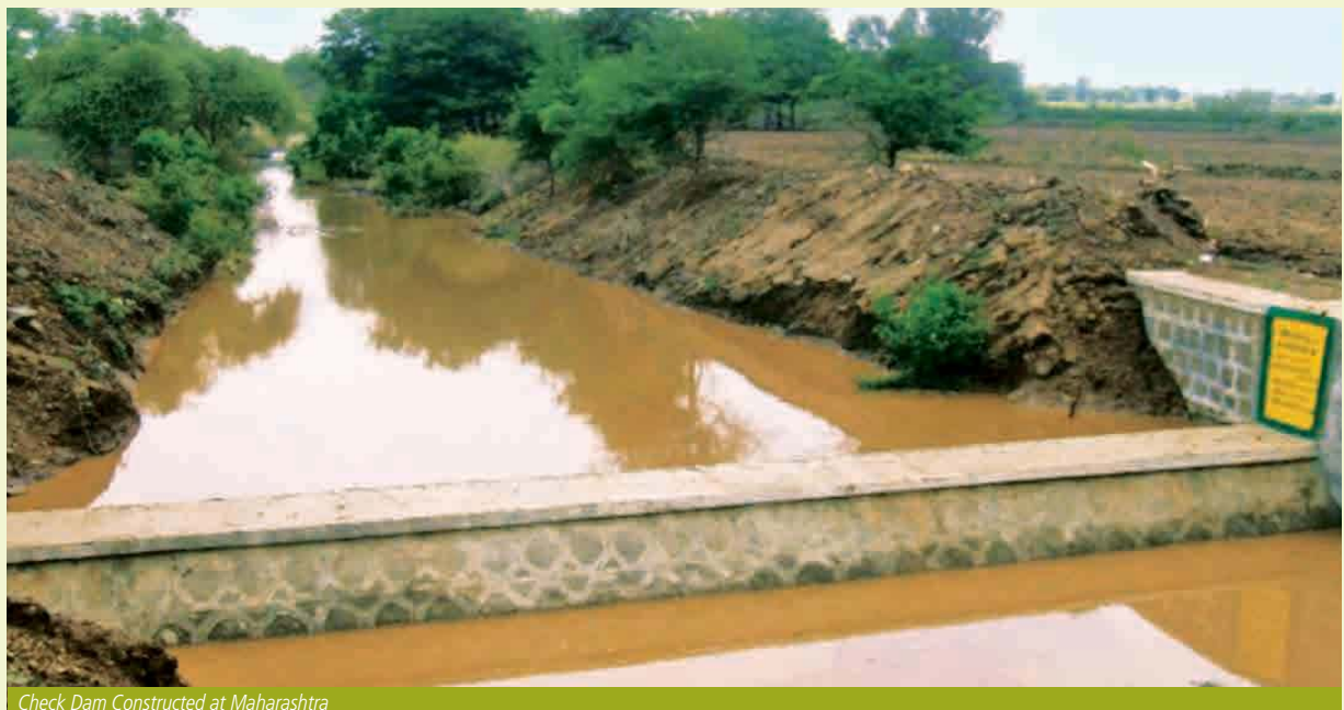
Check Dam Constructed at Maharashtra
