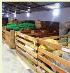
Cable drum wood is used for making partition walls in stores
