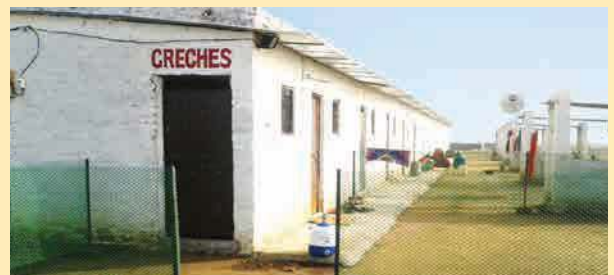
Crèche facility for children of workmen
