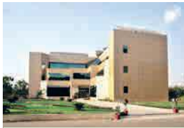
Administrative Building, LTSSHF, Hazira
