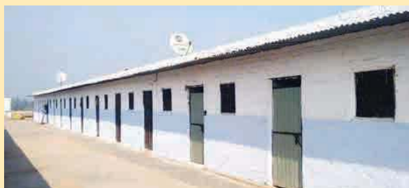
Comfortable accommodation at Workmen's Camp
