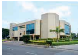
SBU Block (2nd floor), Hazira
