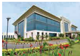
Administrative Building, Vadodara
